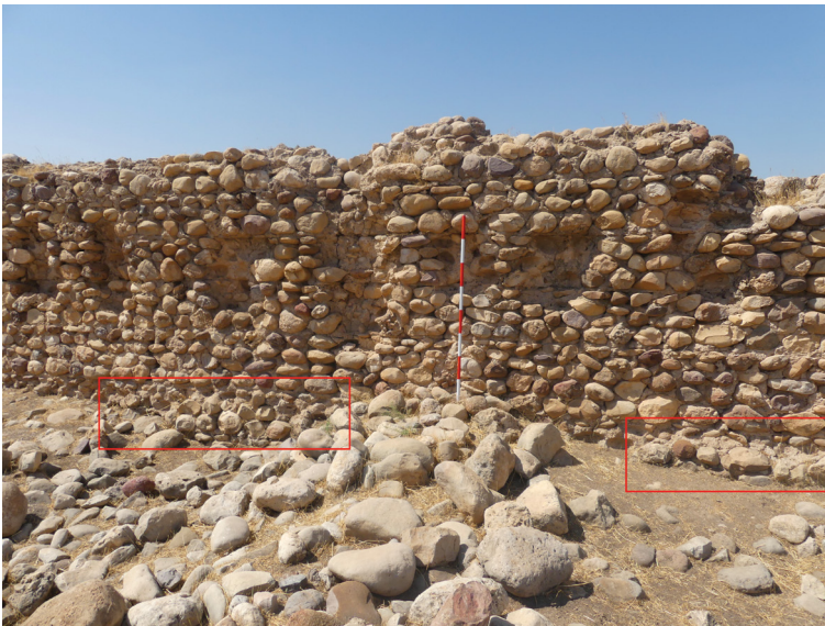
Figure 7 Masonry of the western external wall
