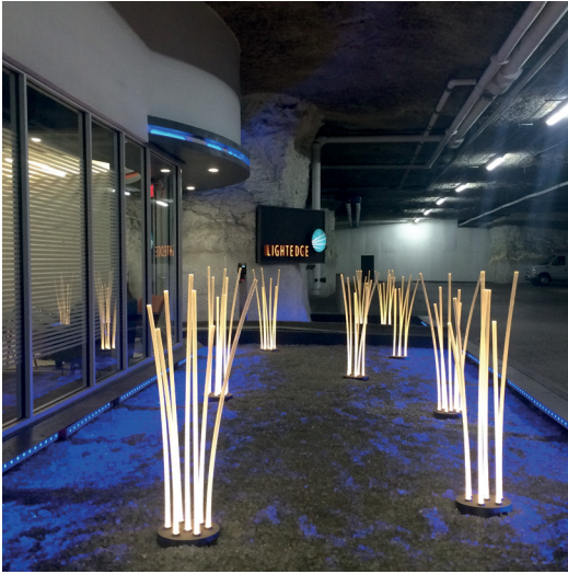
Figure 2 In 2014 Light Edge Solutions opened a digital co-location centre inside of a former limestone quarry in Kansas City, Missouri. Photograph by the Author
