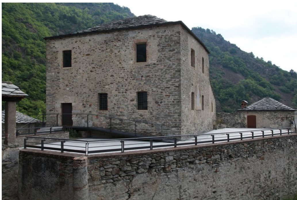
Fig. 7 – Quart, Castello, mastio
