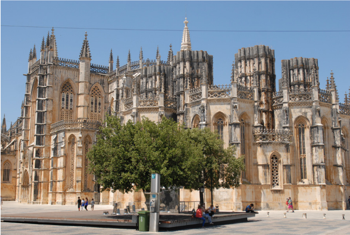
Figure 2a View of Royal Monastery of Batalha
