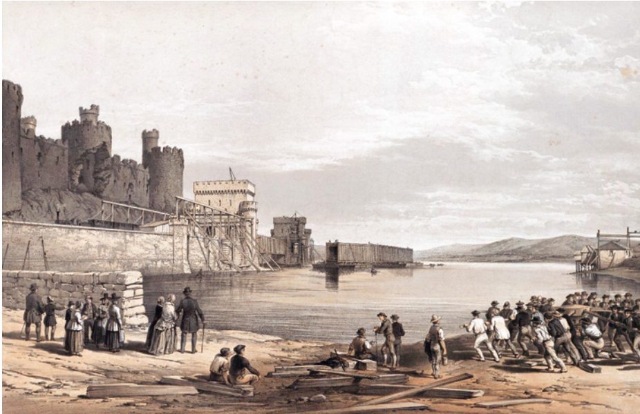
Figure 15 George Hawkins, Lithograph showing the second wrought-iron box girder tube of Robert Stephenson's tubular railway bridge at Conwy being floated into position (September 1848), 300 × 465 mm (image), 370 × 547 mm (paper). Impression digitized by National Library of Wales. © Wikimedia Commons
