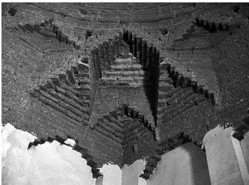
Fig. 29. Detail of one of the splays of the emāmzāde. (Photo: Rudy Favaro ).
