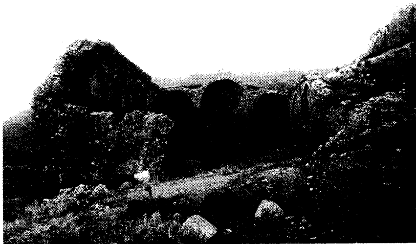
1. View of church ruins from the south.
