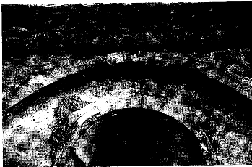
5. Remaining decoration above arch opening on west wall.
