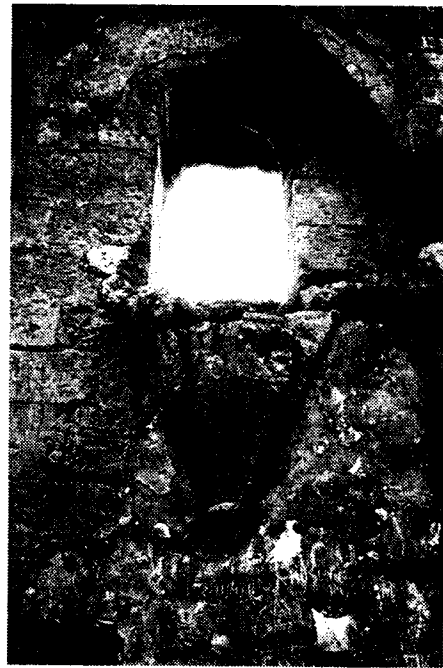
8. West wall balcony support and arch opening.
