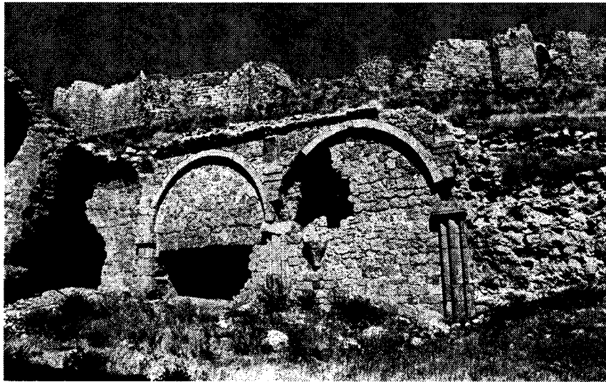
3. General view of east wall.
