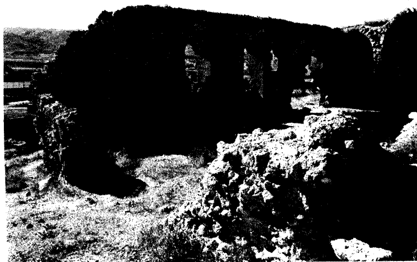
2. General view of west wall.
