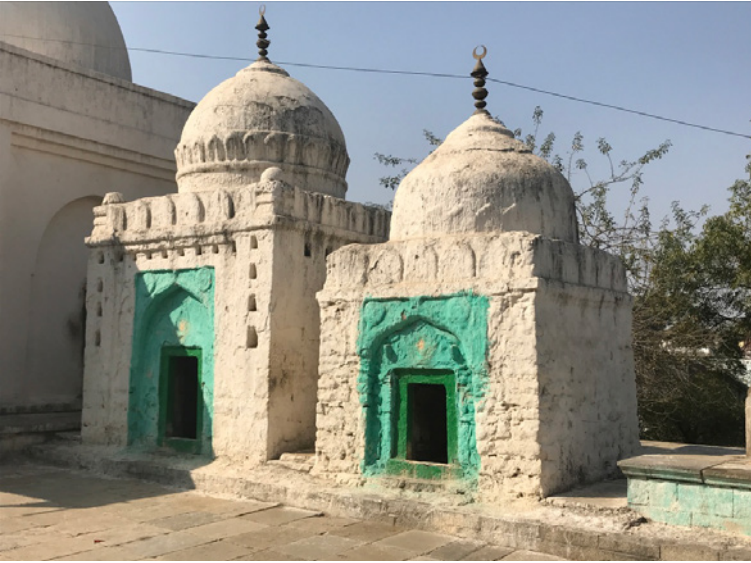
Figure 11 Minor structures in the 'Allama Prabhu temple' in the village of Madiyal. Photo by Sara Mondini
